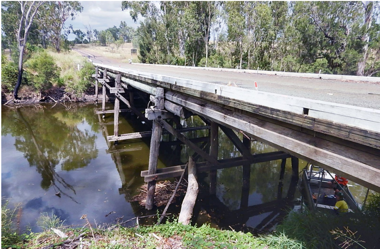
Inspection work being carried out on the Gogango Creek bridge.
