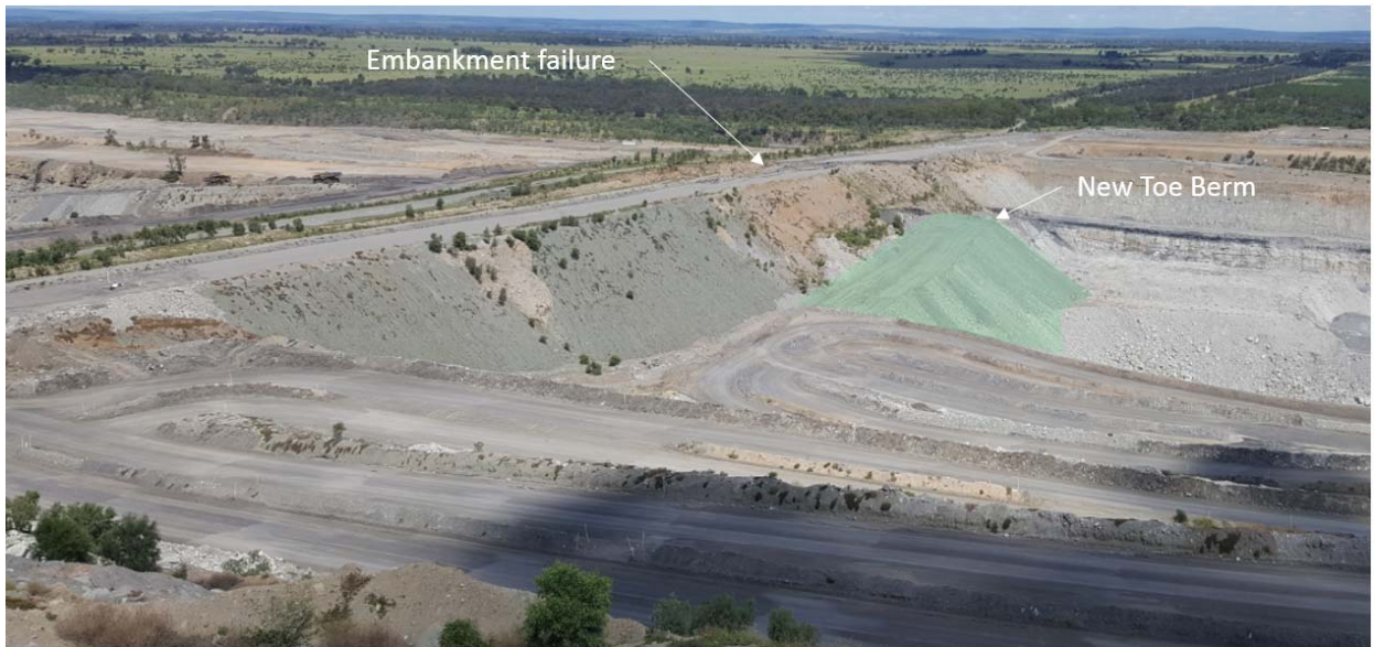
Figure 1 Newly Installed Toe Berm
