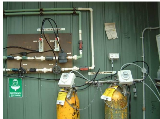
Photos of Chlorine System Installation
