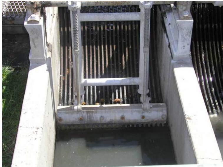
Figure 5.1: Automatic rake collecting screenings from bar screen
