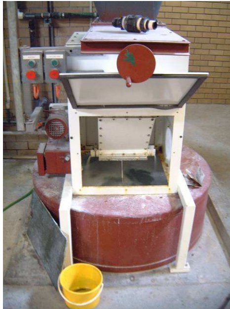
Photo of Alum Screw Feeder and Dilution Tank
