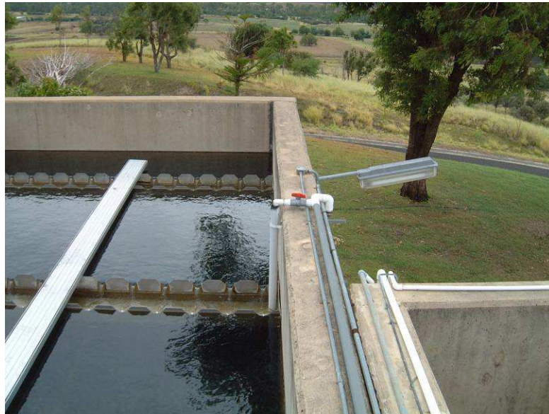
Photo of Temporary Clarifier Access Board
