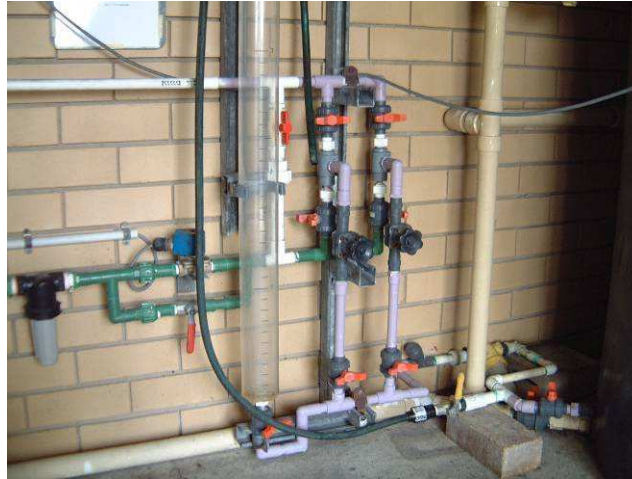
Photo of Polyacrylamide Dosing Eductors
