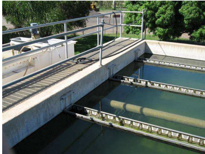
Photo of Railings Around Clarifier
