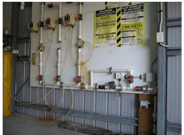
Photos of Chlorine Dosing System
