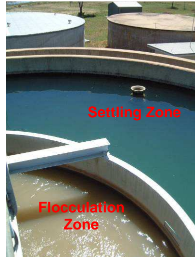
Photos of Stage 2 Clarifier Showing Central Flocculation Well and Settling Zone
