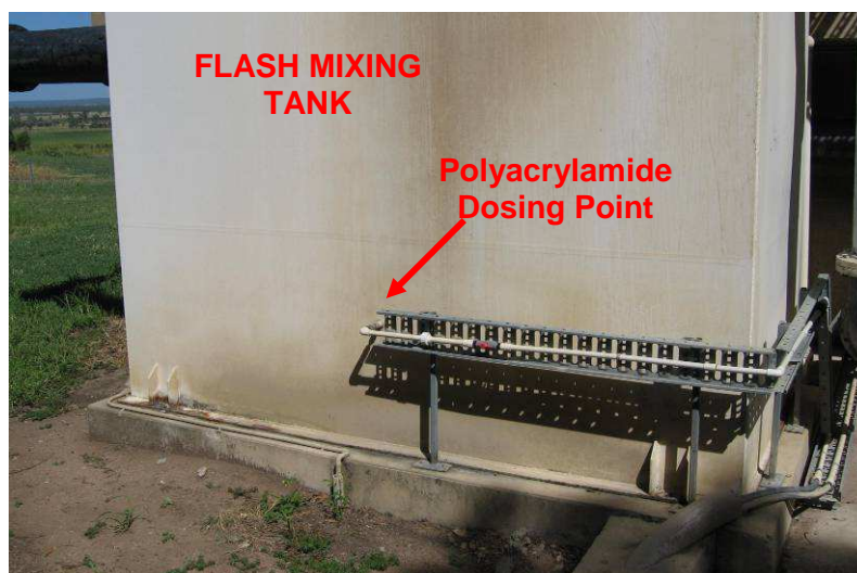
Photo of Polyacrylamide Dosing Point in Flash Mixer
