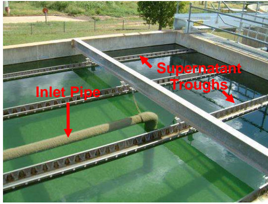
Photo of Stage 1 Clarifier
