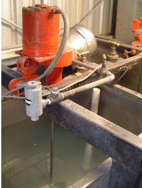
Photo of Polyacrylamide Makeup Eductor and Mixing Tank
