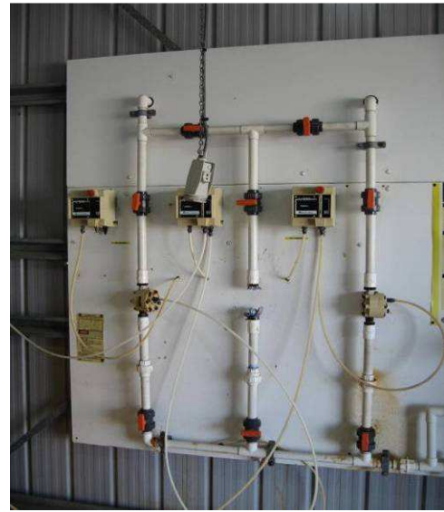
Photos of Chlorine Dosing System
