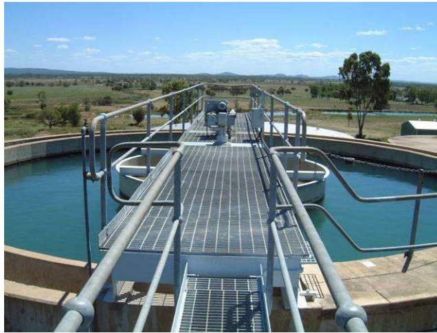
Photos of Stage 2 Clarifier Showing Central Flocculation Well and Settling Zone
