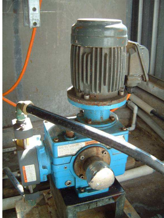
Photo of Polyacrylamide Dosing Pump
