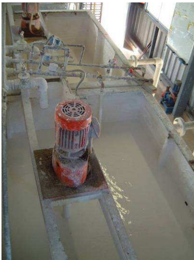
Photo of Lime Tank and Mixer
