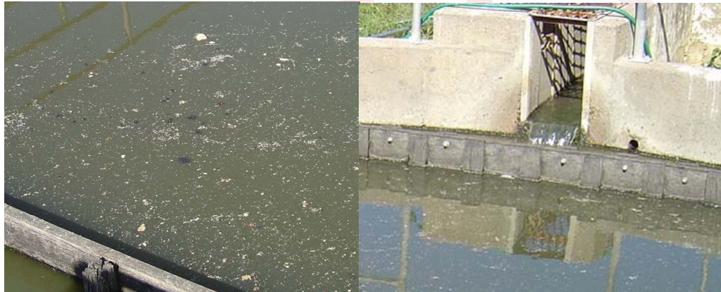
Figure 5-2: Imhoff Tank
