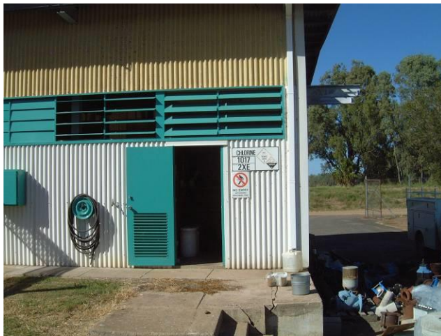
Photo Showing Chlorine Room Door
