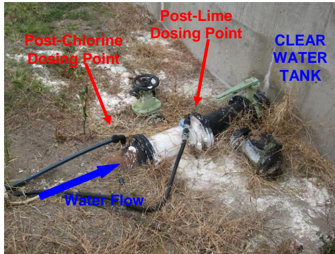
Photo of Post-Filtration Chemical Dosing Points
