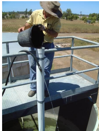
Photo of PAC Dosing to Filter Bed
