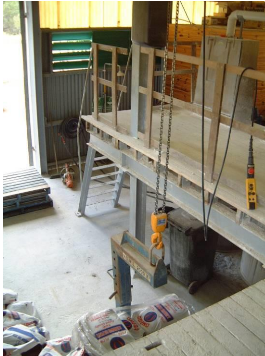
Photo of Bag Unloading Platform for Alum and Lime
