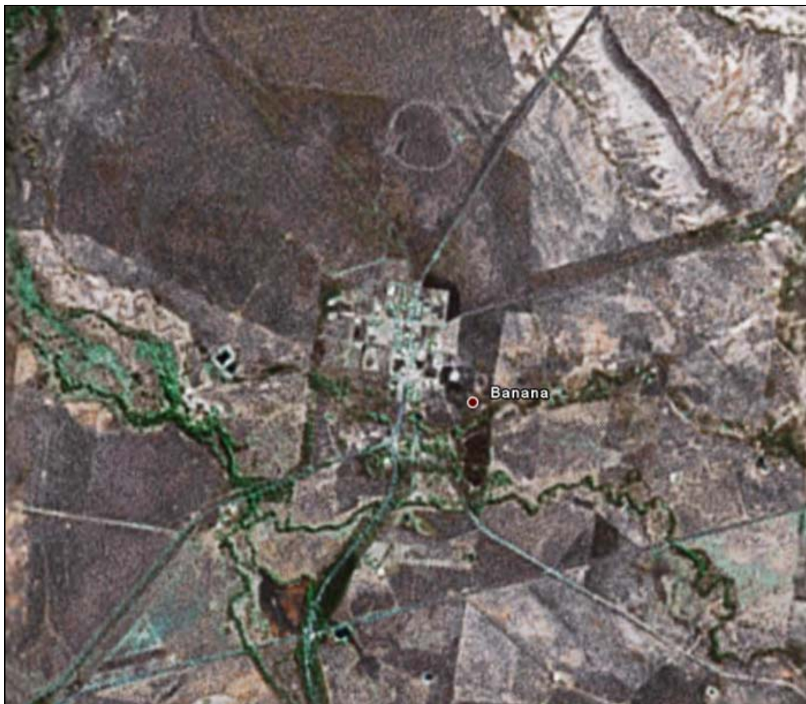
Figure A2 – Aerial Photograph of Banana
