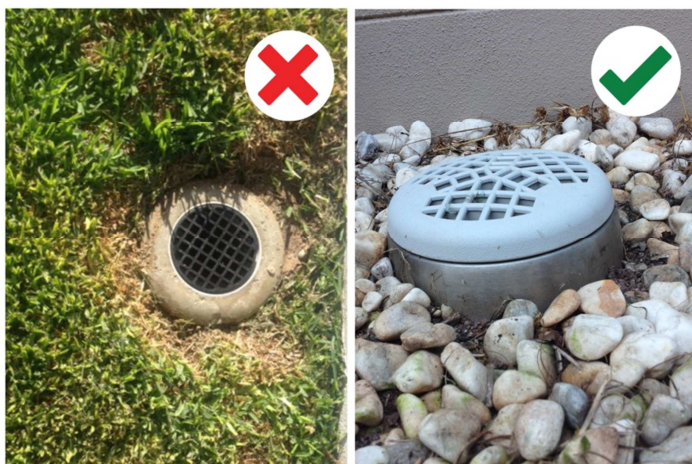
Incorrect and correct way of ORG installation
