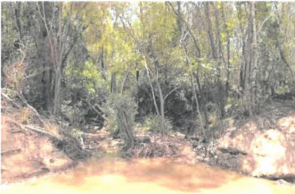
Photo B Looking downstream (after waterway barrier works)
