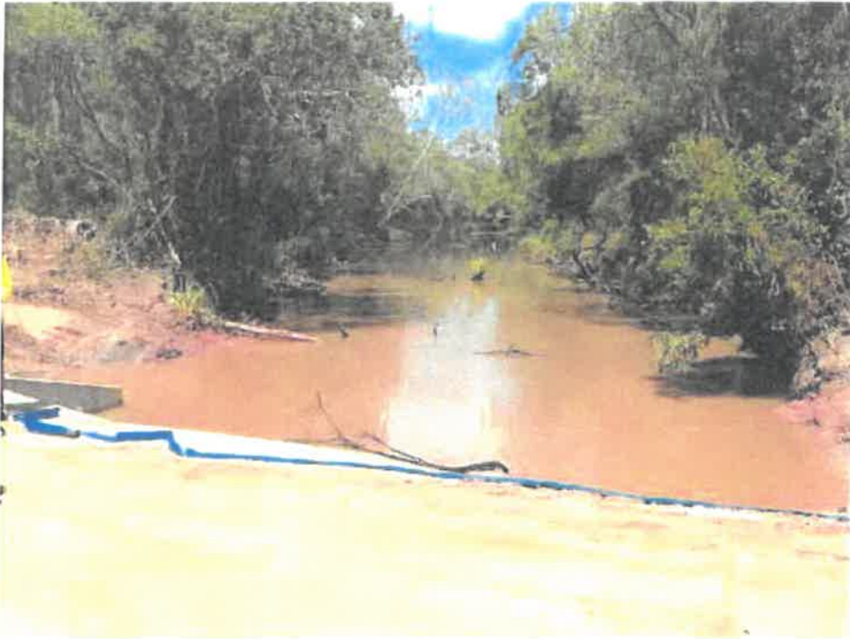
Photo C Looking upstream (after waterway barrier works)
