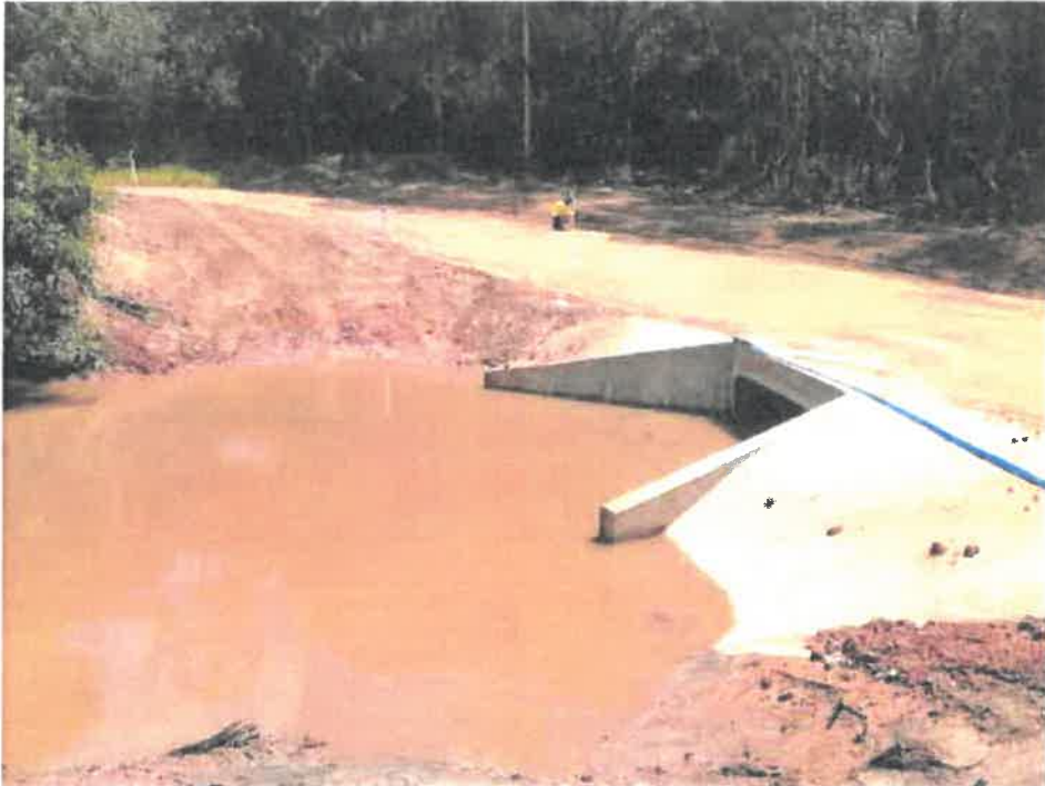
Photo E Looking at the completed waterway barrier works from an upstream position
