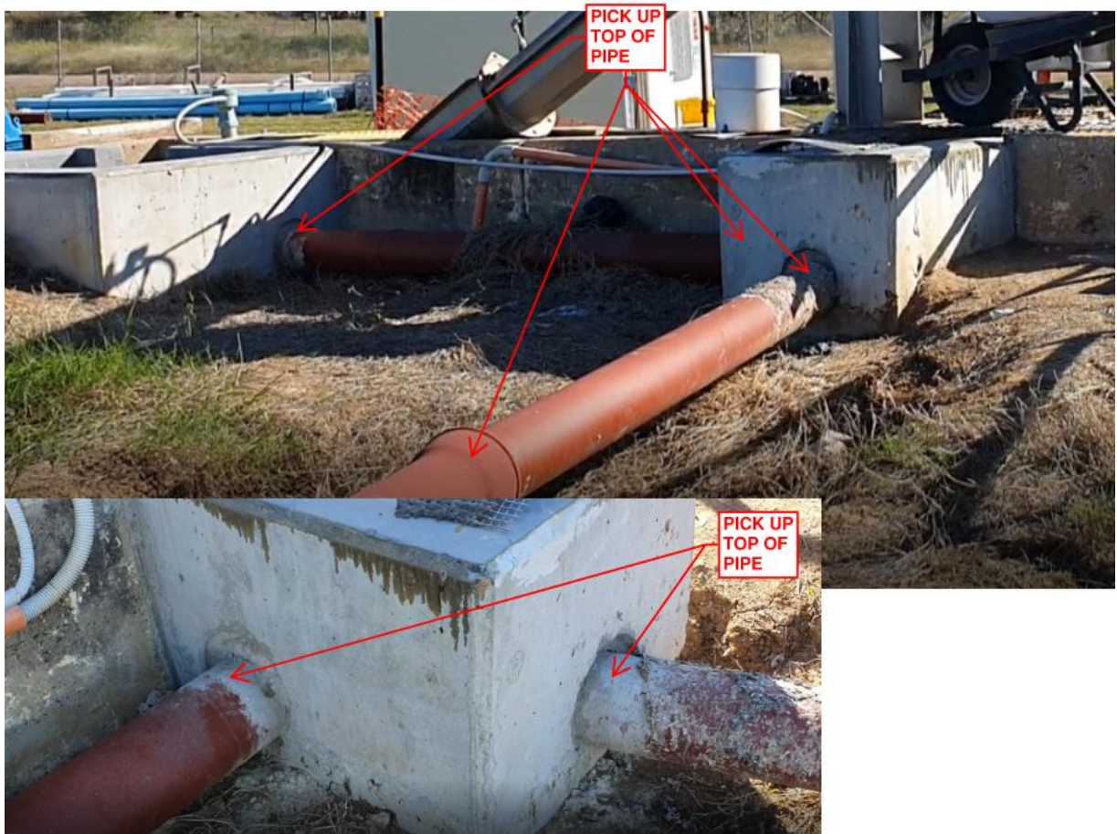
Figure 9 – Critical Inlet Works Infrastructure to be Picked Up
