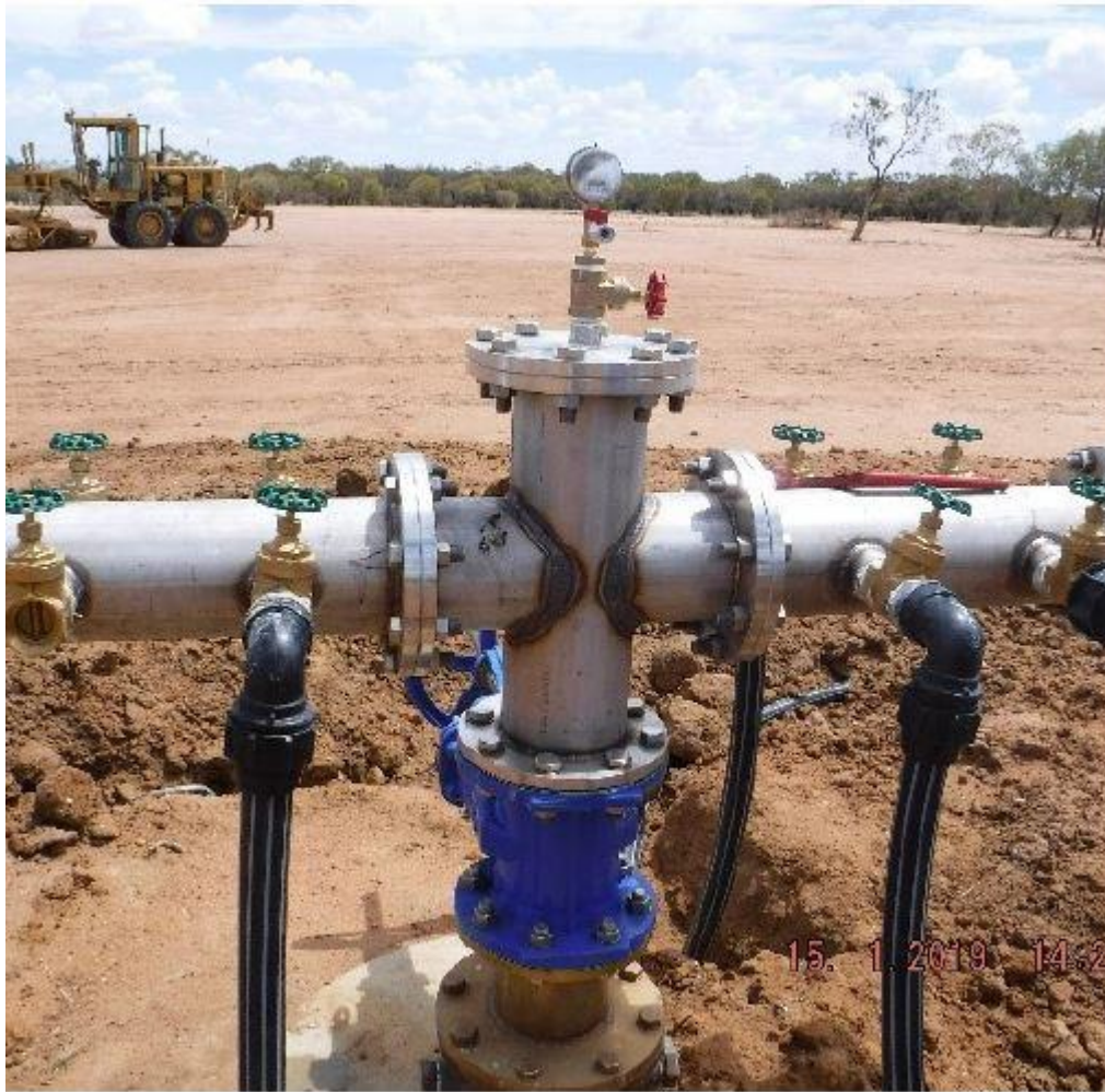
Fig 2 – Slanted Bore Head arrangement
