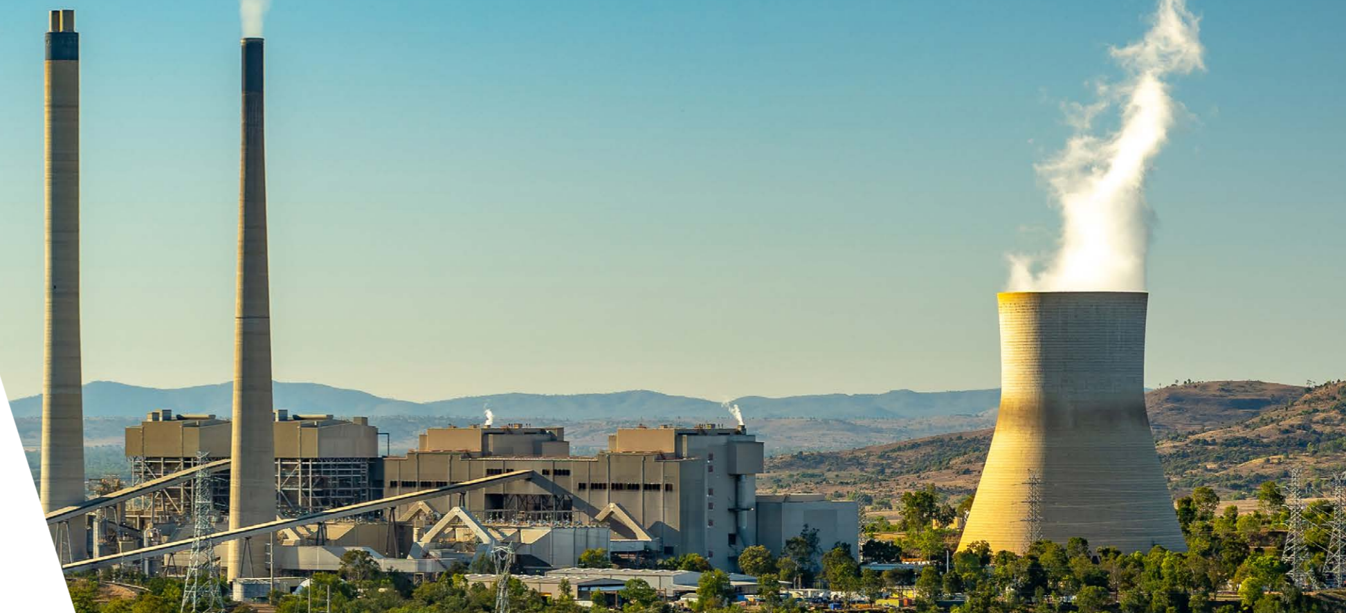
CS Energy Callide Power Station, Biloela
