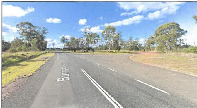
Figure 5: Burnett Highway – Hibbs Road Intersection (Google Street View August 2022)
