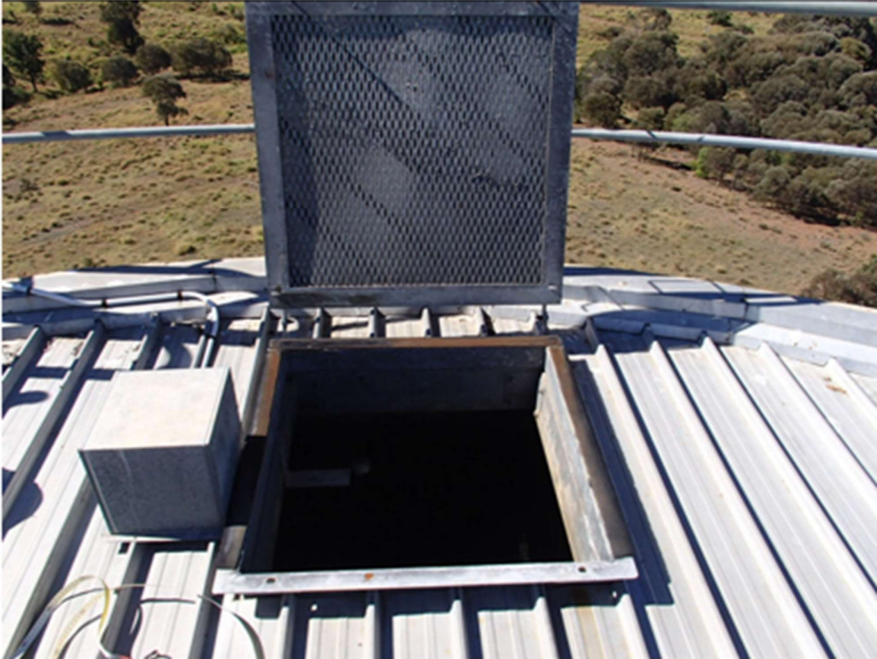
Photos of Reservoir, the Roof and Access Hatch
