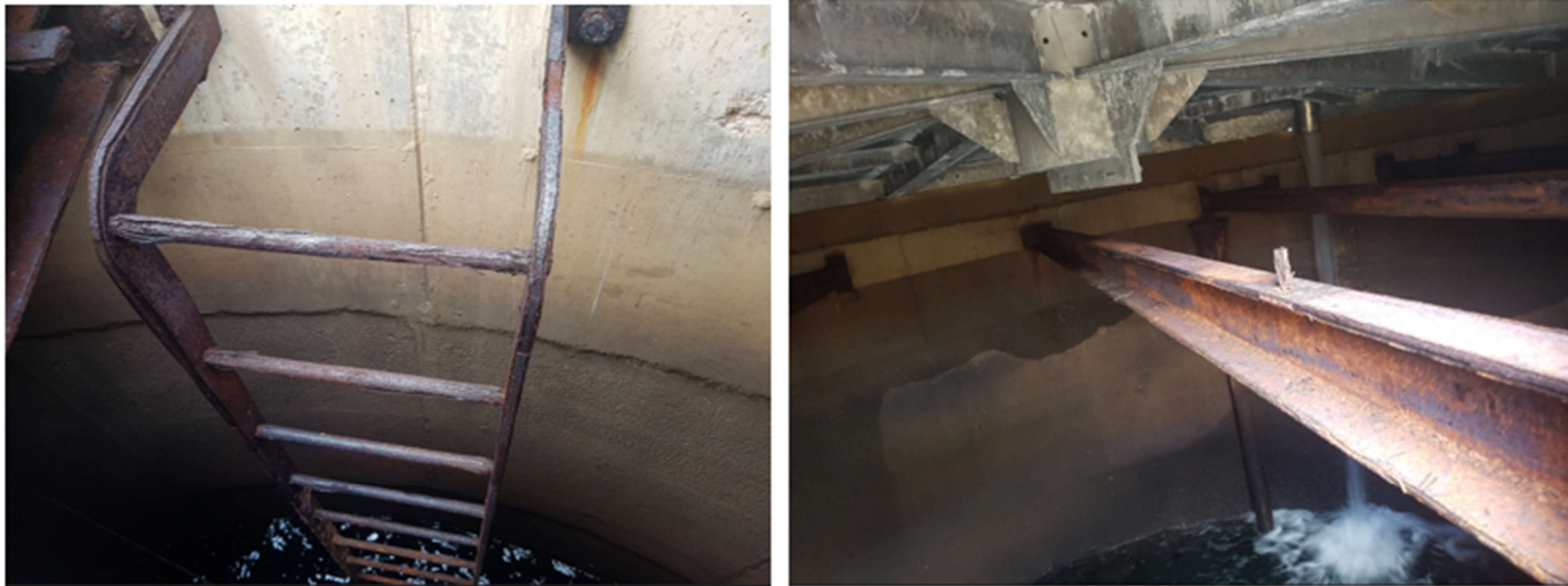
Photos Baralaba Standpipe, Old ladder, and Old Roof Beams
