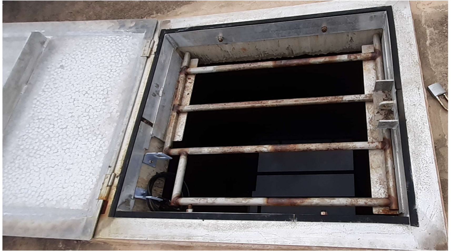
Photos of Reservoir and the Access Hatch
