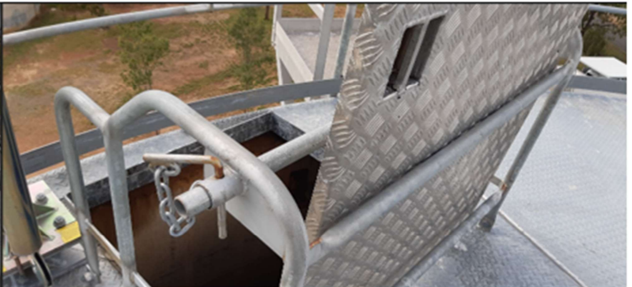
Photos Low Zone Standpipe New Roof and Access Hatch
