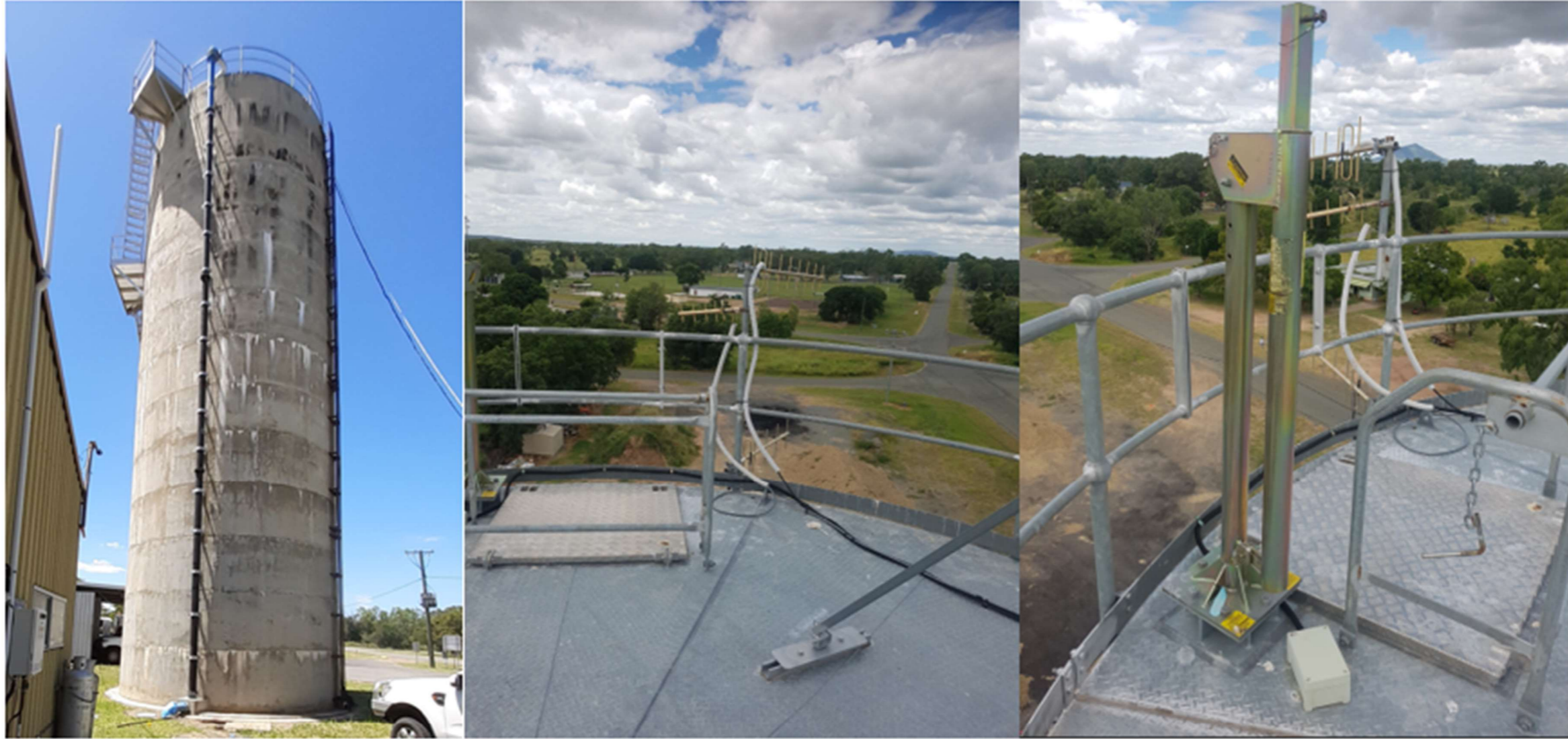
Photos Baralaba Standpipe, New Roof, and Access Hatch
