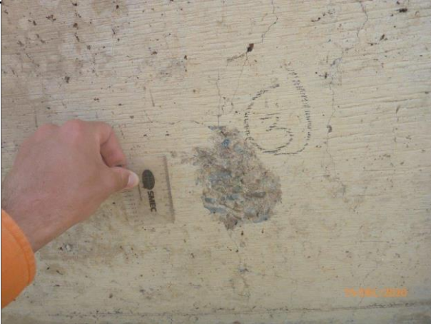
BTF 1 - Repair No. 3
