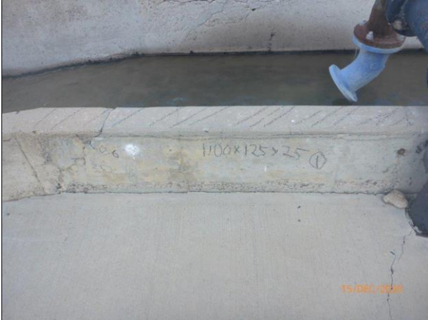
Inlet Channel - Repair No. 1
