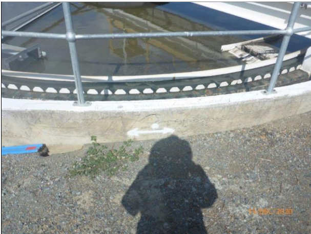
PST 1 - Repair No. 1
