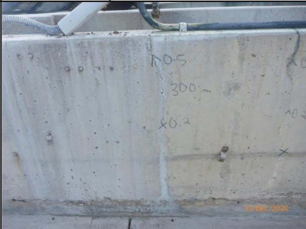
Inlet Channel - Repair No. 10
