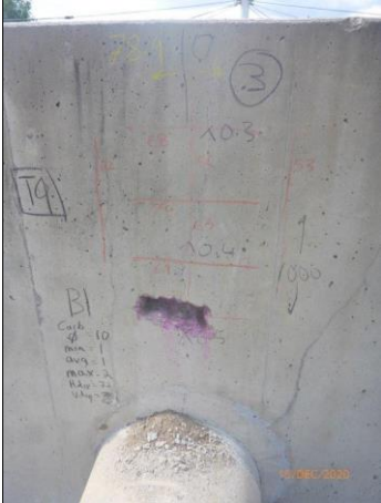
BTF 3 - Repair No. 1
