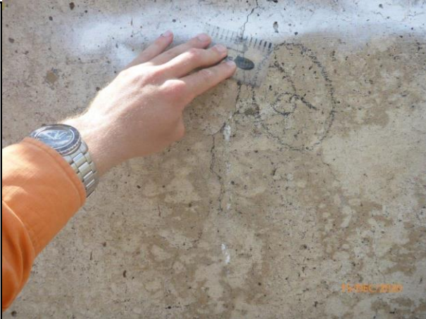
BTF 1 - Repair No. 2
