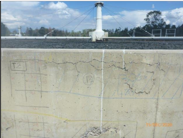
BTF 1 - Repair No. 13
