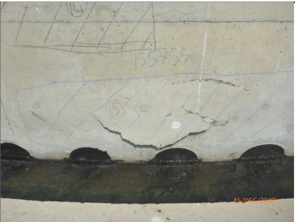
BTF 1 - Repair No. 15
