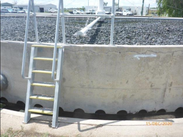
BTF 1 - Repair No. 1
