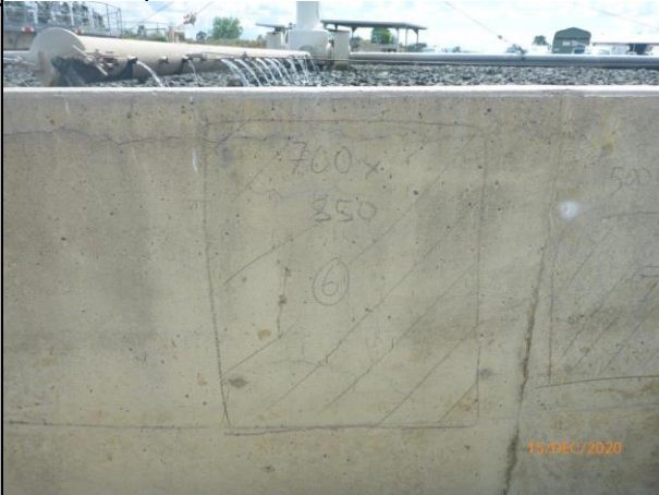
BTF 1 - Repair No. 6
