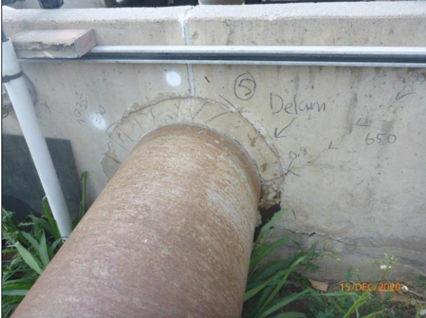
Inlet Channel - Repair No. 5
