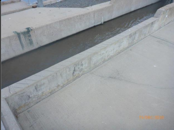
Inlet Channel - Repair No. 2
