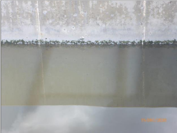
CCT - Repair No. 1
