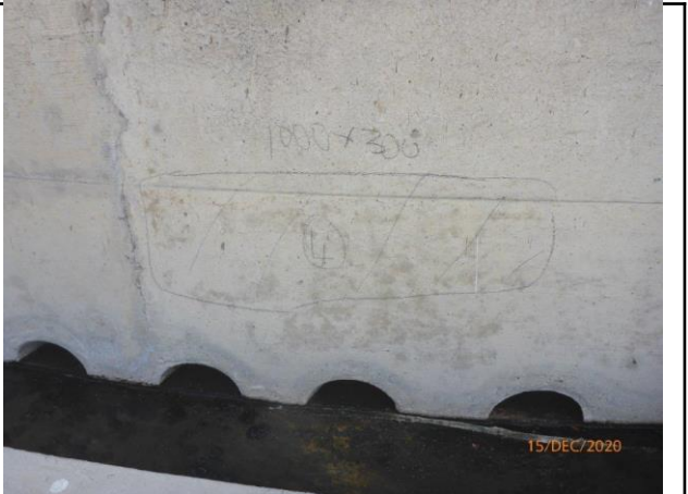
BTF 1 - Repair No. 4
