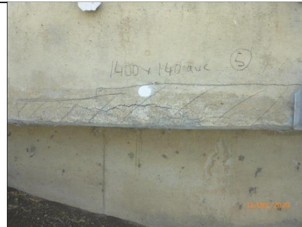
PST 1 - Repair No. 4
