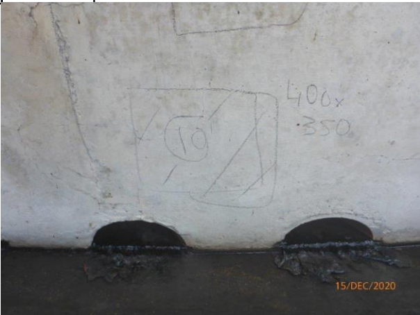
BTF 1 - Repair No. 10
