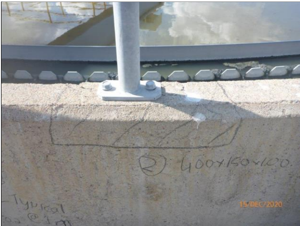
PST 2 - Repair No. 1
