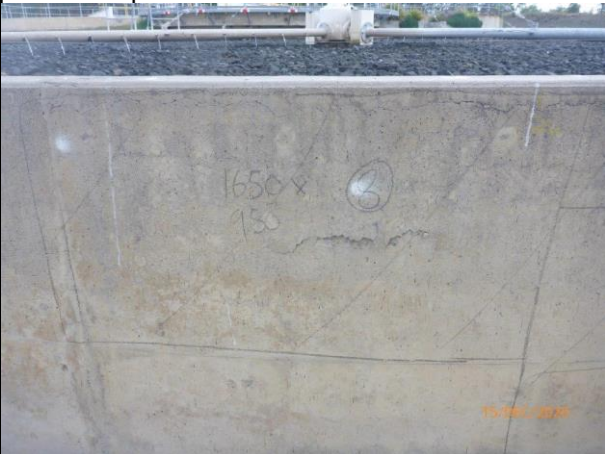
BTF 1 - Repair No. 8
