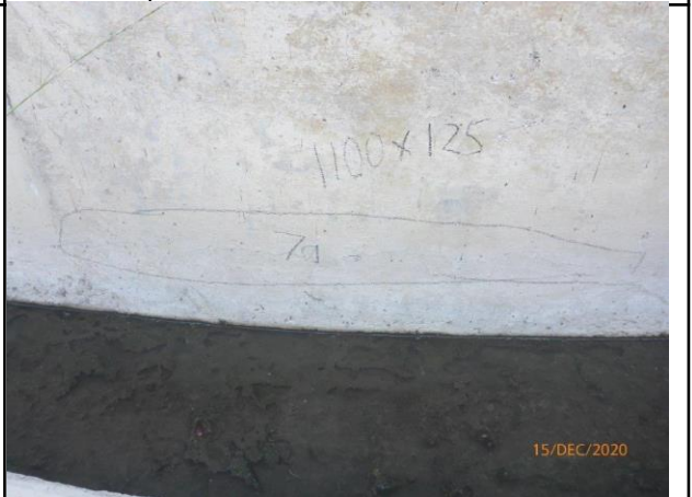
BTF 1 - Repair No. 7a
