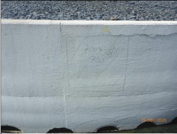
BTF 1 - Repair No. 20
