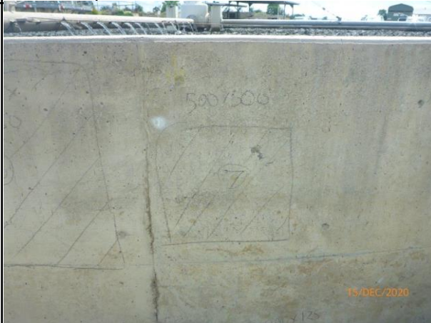
BTF 1 - Repair No. 7
