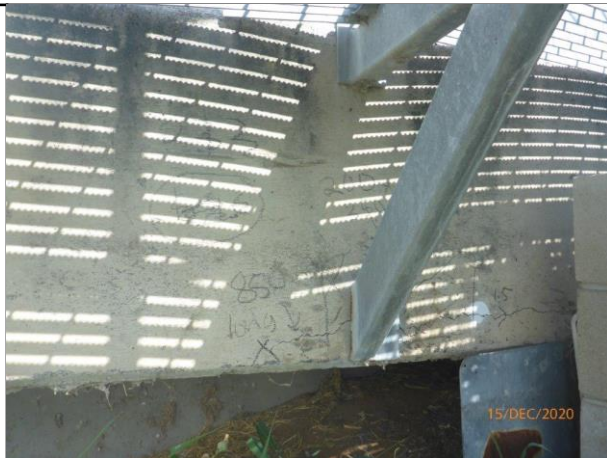
PST 1 - Repair No. 2
