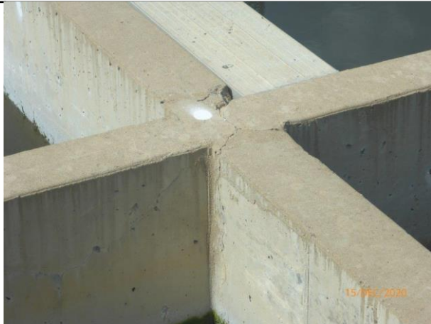
CCT - Repair No. 2
