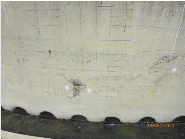
BTF 1 - Repair No. 12
