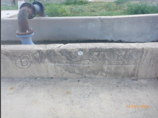
Inlet Channel - Repair No. 6
