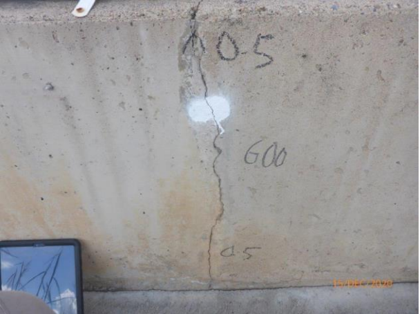
Inlet Channel - Repair No. 8
