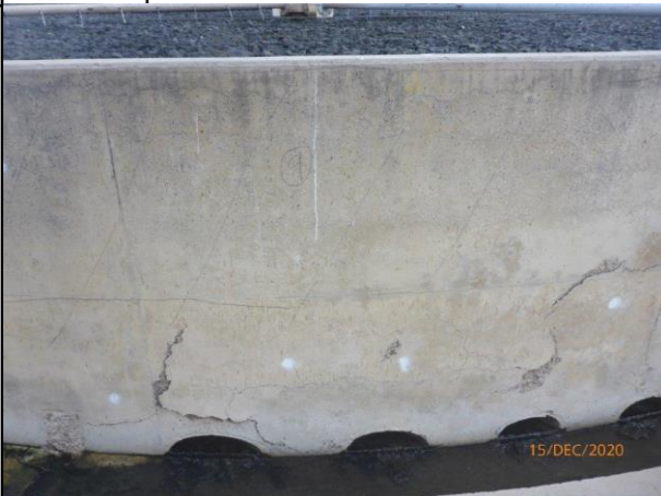
BTF 1 - Repair No. 9
