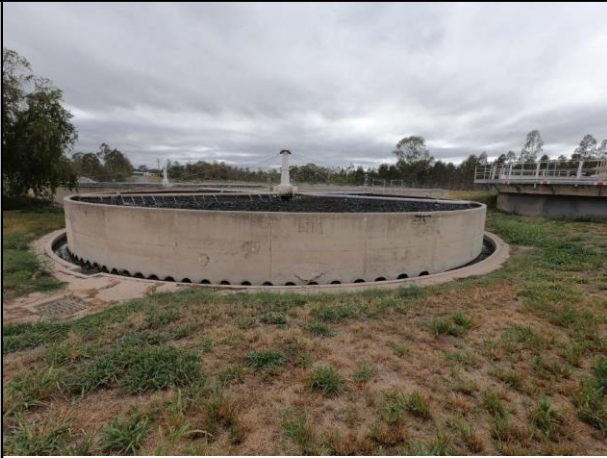
BTF 1 - Repair No. 21
