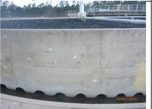
BTF 1 - Repair No. 11
