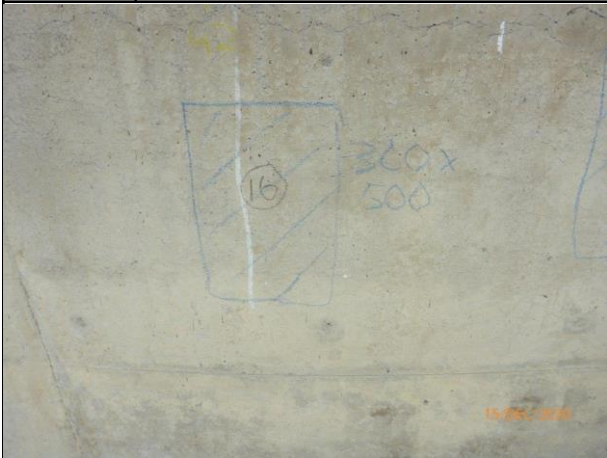
BTF 1 - Repair No. 16
