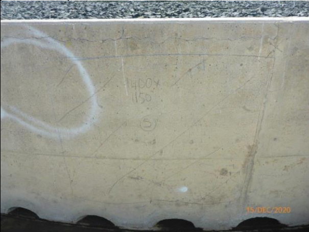
BTF 1 - Repair No. 5
