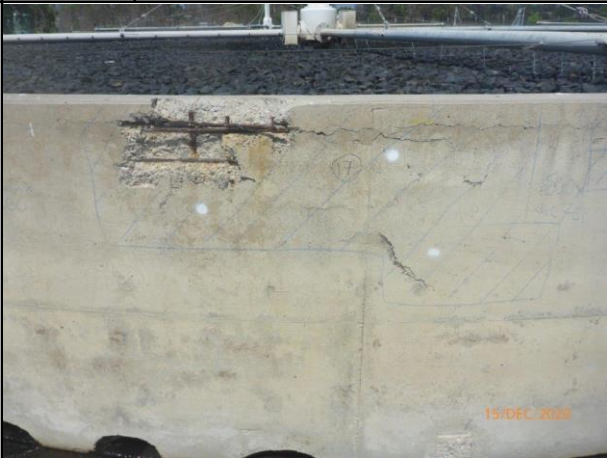
BTF 1 - Repair No. 17
