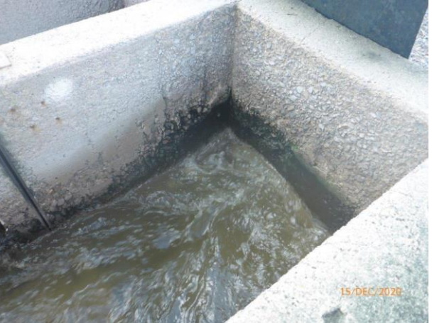
Inlet Channel - Repair No. 7
