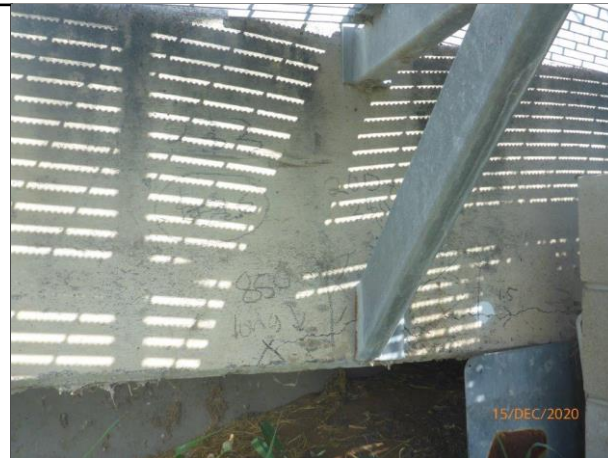
PST 1 - Repair No. 3
