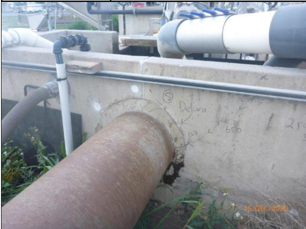
Inlet Channel - Repair No. 9
