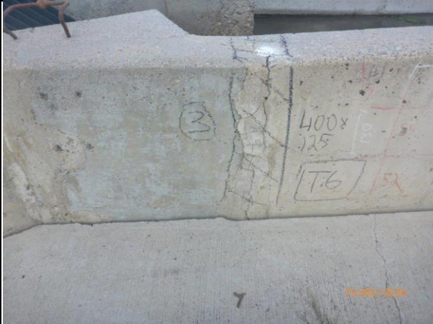
Inlet Channel - Repair No. 3
