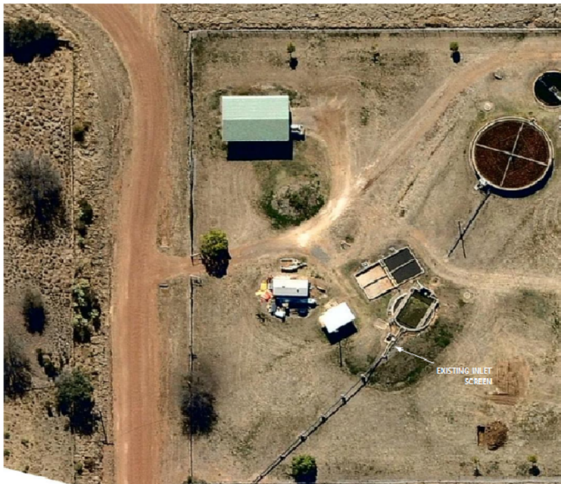
Figure 5-2 - Existing Inlet screen location
