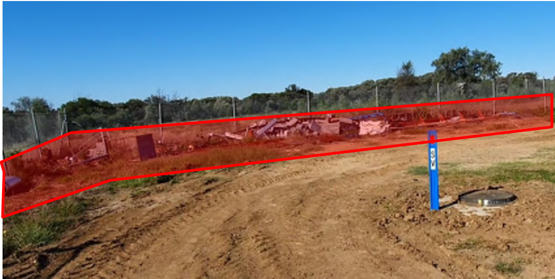
Figure 1 – Stockpiles to Clean – Camera looking East
