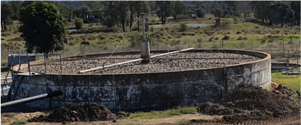
Figure 5-4 - Biological Trickling Filter
