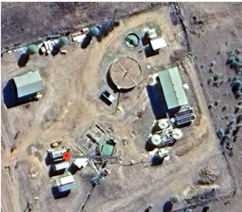
Figure 2-1 – Aerial view of Taroom STP
