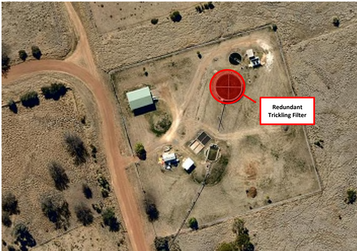
Figure 3 – Taroom STP Site (prior to the recent upgrade works)
