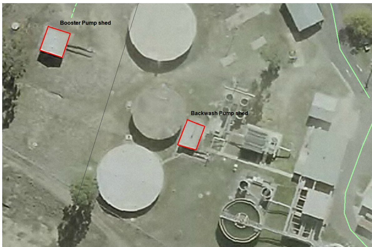
Fig 1 – Moura water treatment plant
