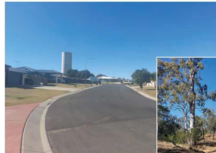
Pictured: Earlsfield Street Drainage and Pavement Upgrade, Biloela
