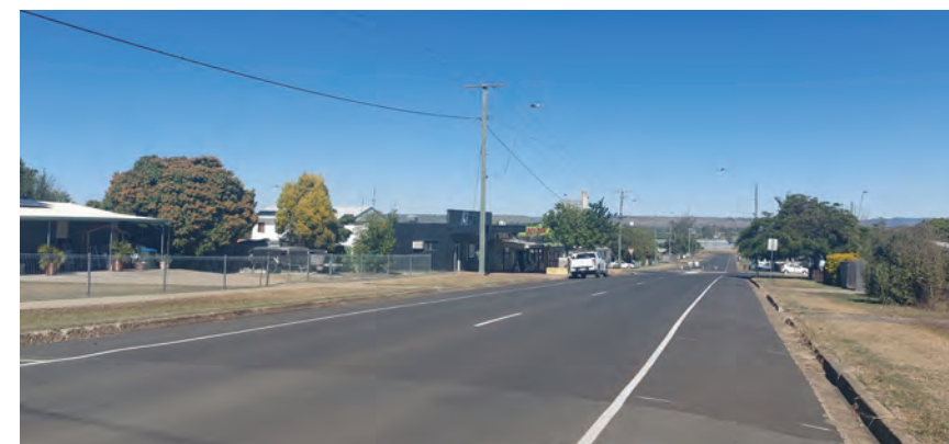
Pictured: Washpool Street Reseal, Biloela
