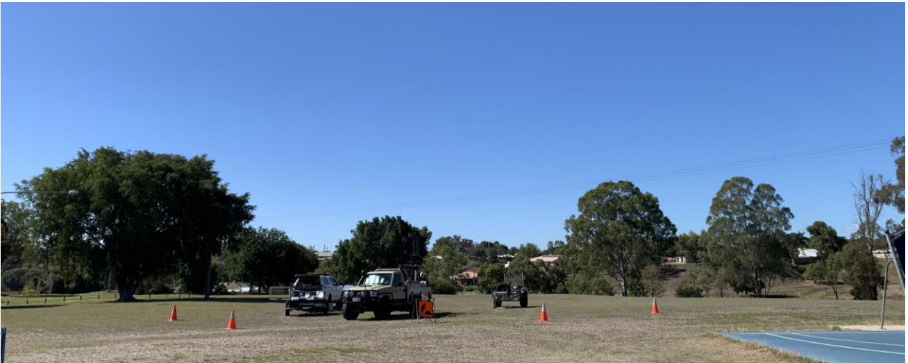
Photograph 2: Looking north towards borehole BH4.
