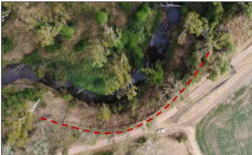
Figure 2 – Plan view of site showing extent of the erosion
